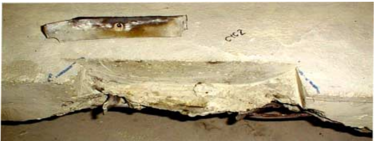
Figure 8. Condition of concrete surrounding the connector after completion of cyclic test #2.
