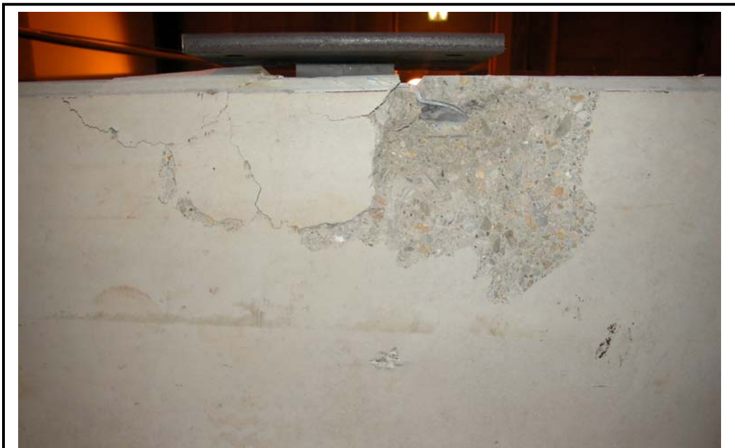
Figure 35: Bottom View of Slab
